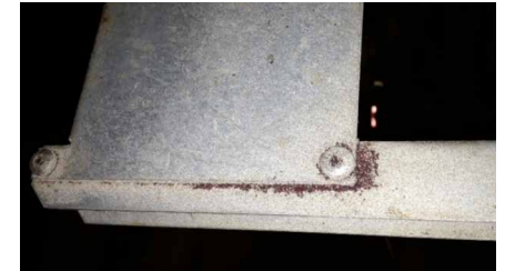
Typical mite "nest" in a screwed joint
